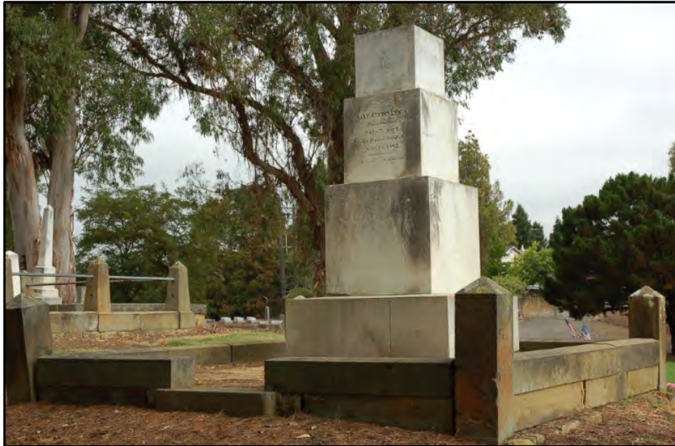
Photo 13. Pioneer Section, Lynch plot, facing northwest.
