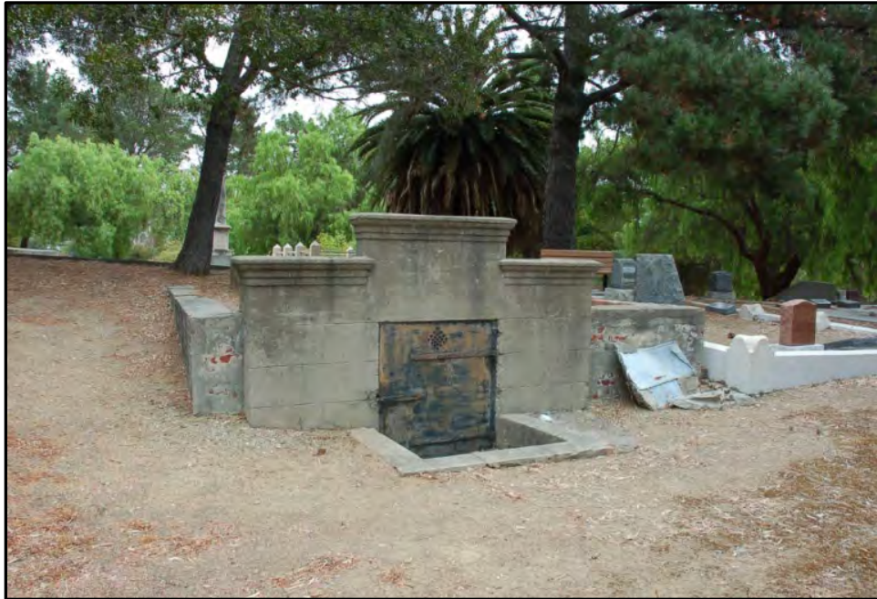
Photo 11. Central Section, Thomas T. Hooper vault, facing northeast.
